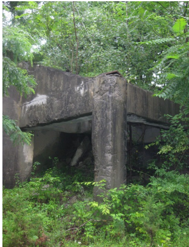
Figure 27. Photo of concrete foundation (c. 1937) of crusher used to reduce cement stone for use at Universal Atlas' cement plant in Greenport, New York.
