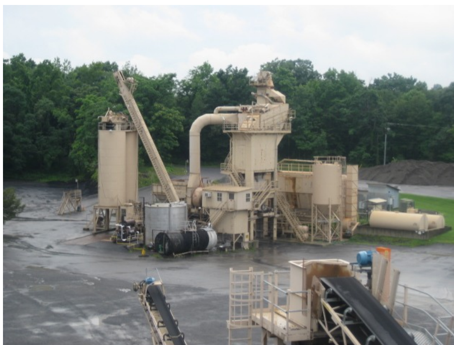
Figure 20. Photo showing blacktop plant at Colarusso quarry on Becraft Mountain.
