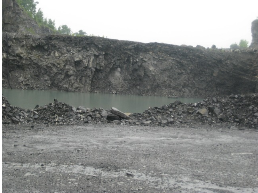
Figure 11. Photo of the north face of Mower's Lake showing the complex folding and thrust-faulting typical of this quarry. The dark colored rock at the upper right of the face is from the lowest part of the New Scotland Formation. It occurs in a sheet that has been thrust over a complex mélangé of Port Ewen-Alsen-Becraft.
