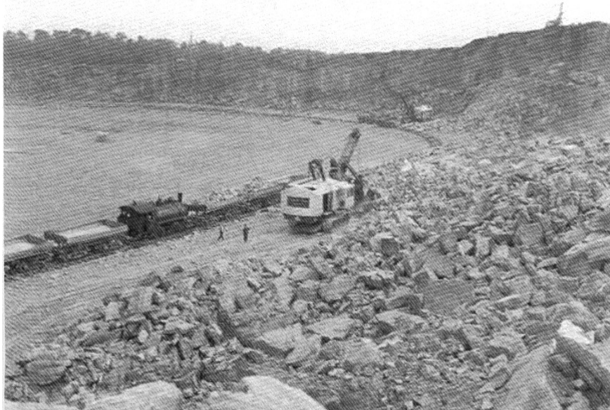
Figure 2. Electric shovel loading rail cars on the floor of the Universal Atlas Greenport Quarry in 1936.
